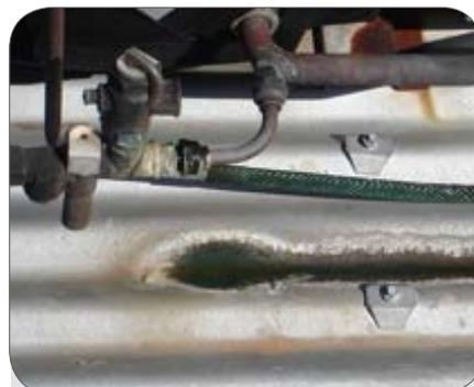
**Figure 1** Bi-metallic corrosion caused by "copper-rich" water run-off
